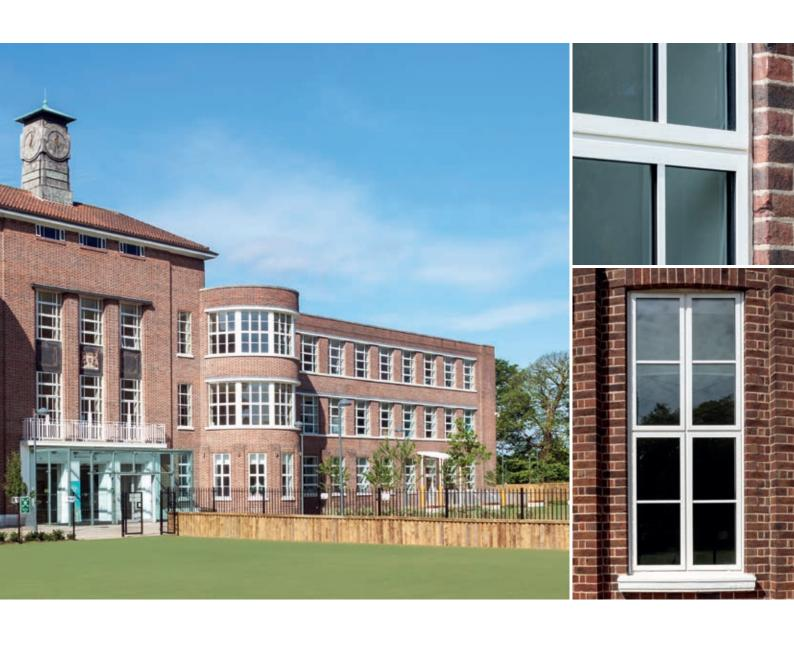
The Alitherm Heritage and Smart Wall systems provided a truly authentic appearance for this sensitive refurbishment project, with the replacement windows having to replicate the original steel fenestration.
